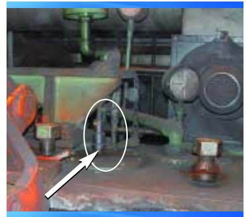
Hyrolert Transducer installed on a bank of rollers at a steel mill facility.
