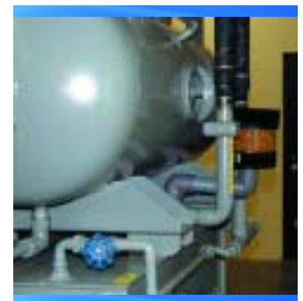
Watchdog Breather installed on a hydraulic reservoir.
